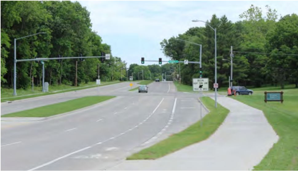
Photo 3.3 - Sidepath trails may be supplemented by an on-street bicycle facility. This allows pedestrians and slower cyclists (e.g. children) to use the sidepath, while faster cyclists may choose to bike on the street.
