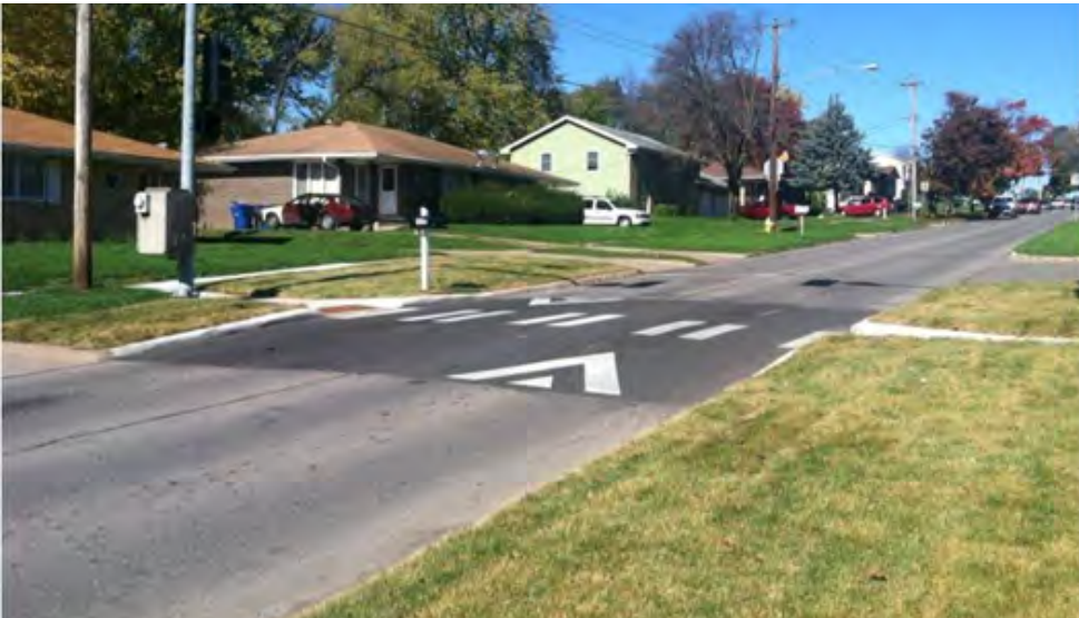
Photo 3.6 - A raised crosswalk slows traffic through vertical deflection and makes pedestrians crossing the street more visible.
