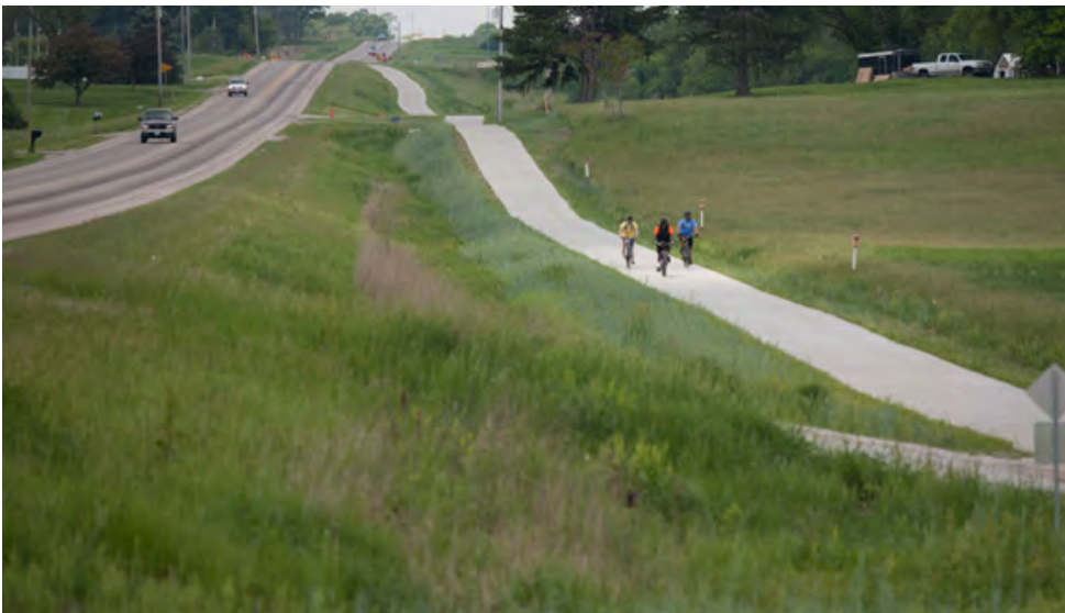
Photo 3.4- Sidepath trails may be appropriate along rural roadways with a few low-volume driveways or intersections.
